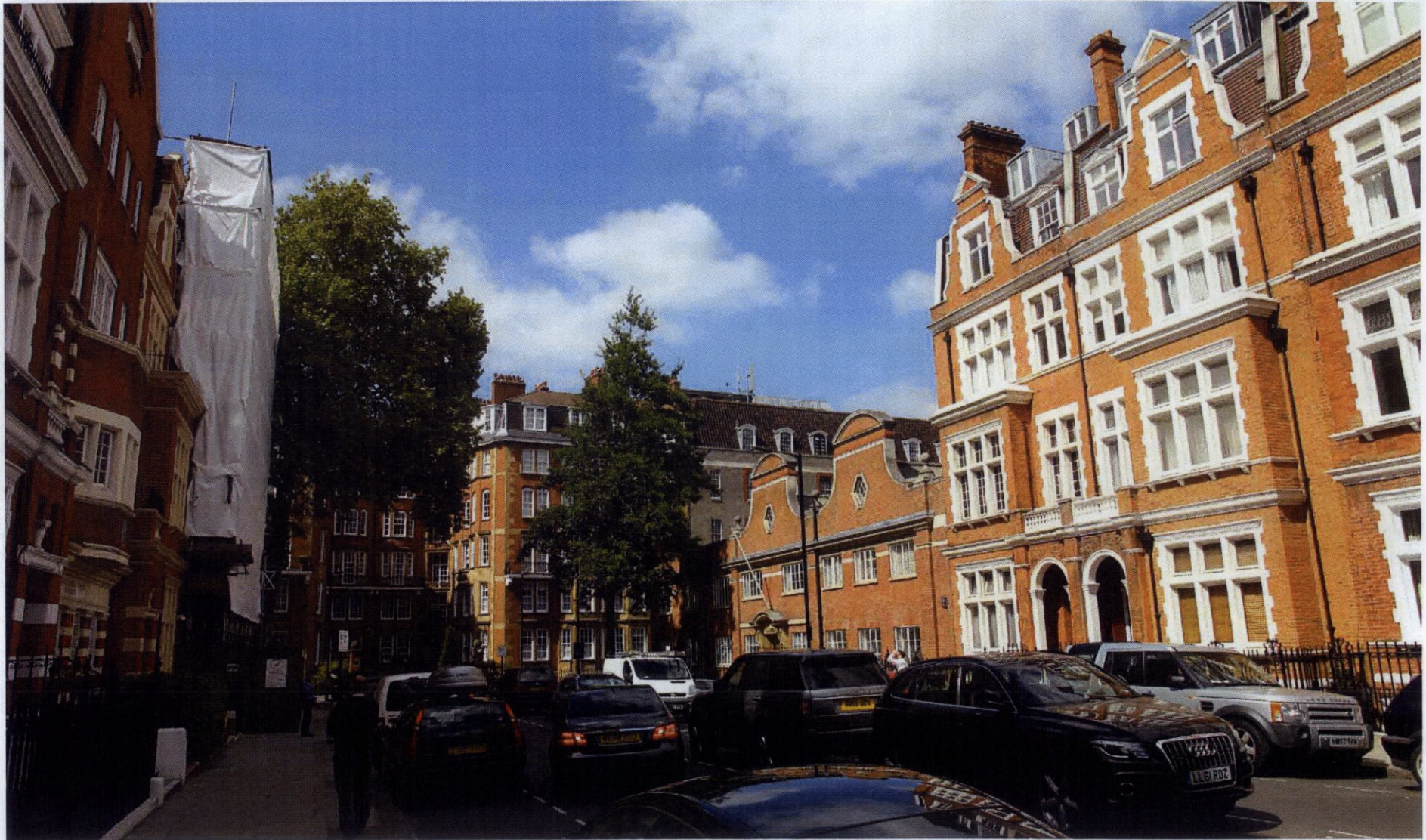
Fig.6.41. Palace Court looking north towards Moscow Road - Existing.
